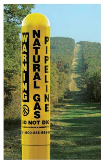
Pipeline marker signs are located at road, railroad, and navigable waterway crossings. These markers identify the approximate location of a pipeline at numerous points along the pipeline right-of-way. Each operator's marker may look different, but the purpose and information on the marker is the same. Markers tell you the:
